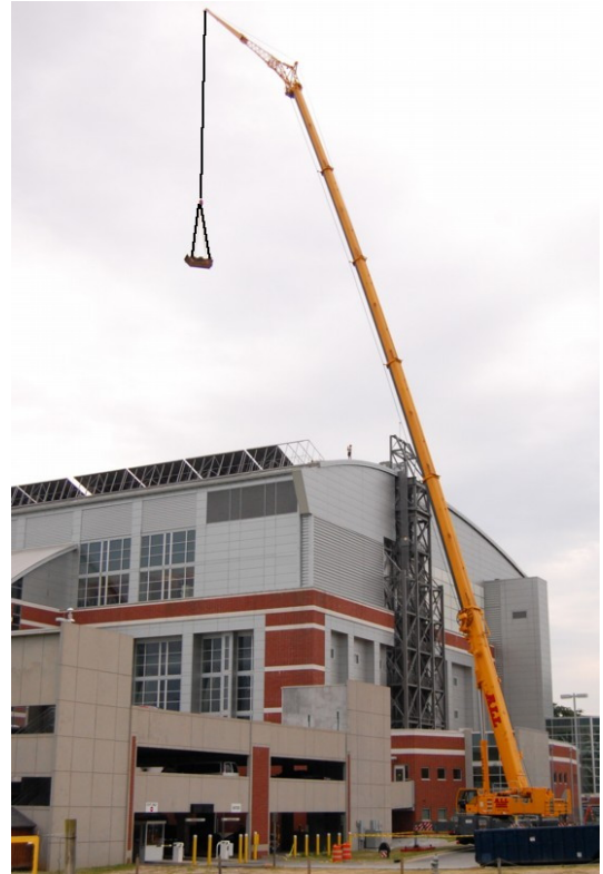
Fig. 1. Telescoping Boom Crane with Attached Jib.
