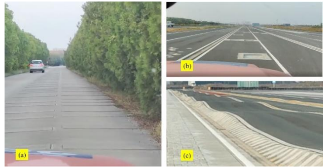
Fig. 7. Photograph of the test road: (a) resonance road; (b) square pit road; (c) undulating road.
